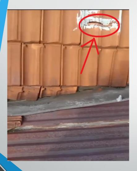
• Failure of previous patch up works on roof tiles and metal deck area as silicone or material used is all wearing out.
