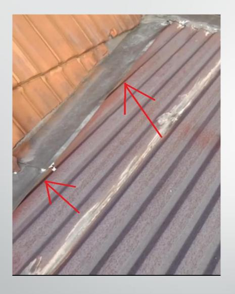
Gaps in Flashing where water can flow thru during heavy wind
