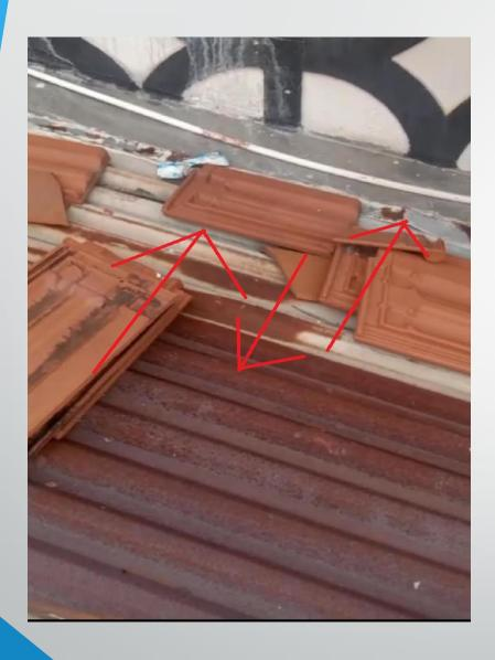
Surface compromised with tiles to hold flashing
