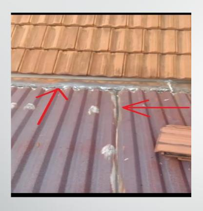
Gaps in roof tiles flashing found.
